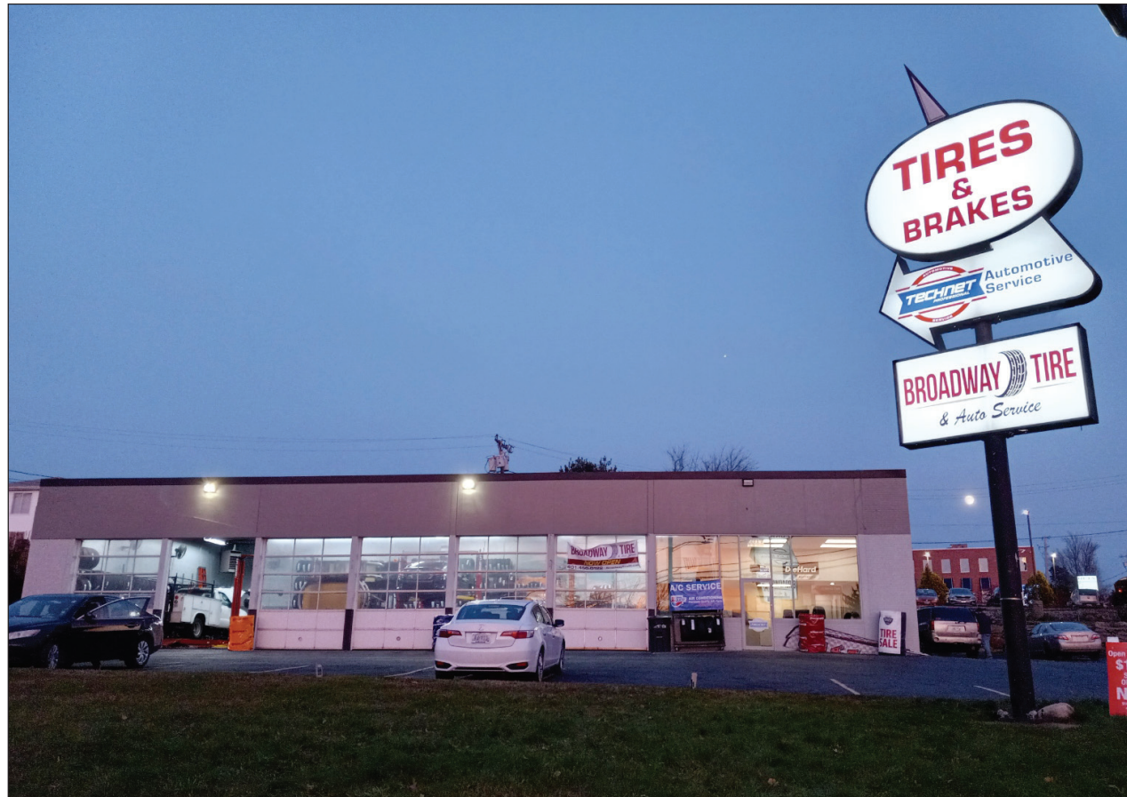
The city of Johnston is proud to feature Broadway Tire & Auto Repair, the third installation of this growing family-run business! Give them a call today at 401-725-3535 for all your tire and auto repair needs.
